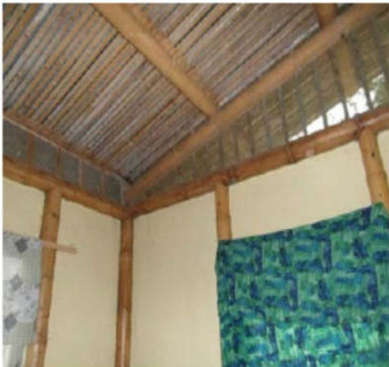
Figure 15: Engineered bahareque housing in Costa Rica.
