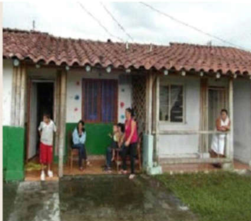
Figure 16: Engineered bahareque housing in Colombia.
