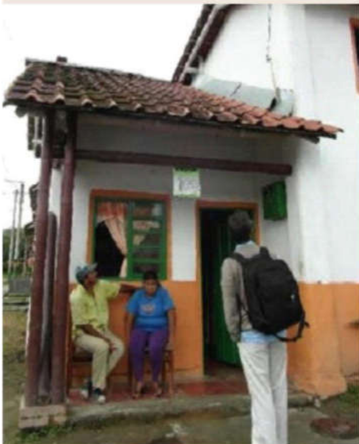
Figure 17: Engineered bahareque housing in Colombia.
