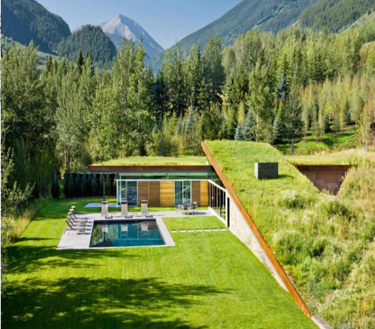
Green roofed Colorado home buried into the earth to save energy, by Lucy Wang
